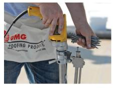
The traditional method for fastening insulation and membrane in low-slope roofing requires roofers to work in awkward, bent-over or kneeling positions, all day, in extreme heat or cold, often for many days at a time; exactly the scenario that can lead to MSDs.
