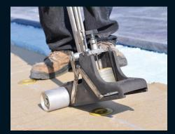
RhinoTrac eliminates over- and underdriving of RhinoBond plates for optimal welding of thermoplastic membranes.
