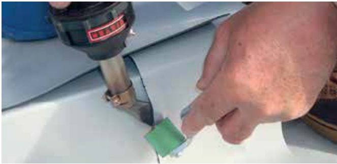
HOT JET S with angled nozzle welding a T-joint on the roof.
